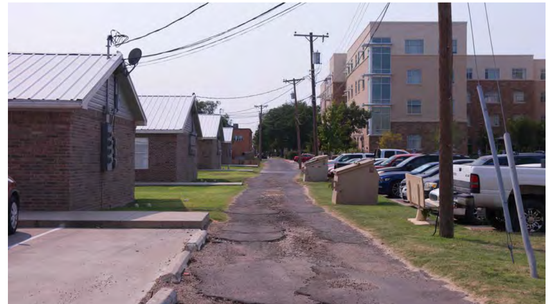
Existing alleyway looking west near 27th
