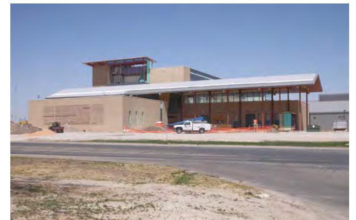
WTAMU continues to build. Agricultural Science Complex under construction in 2017.
