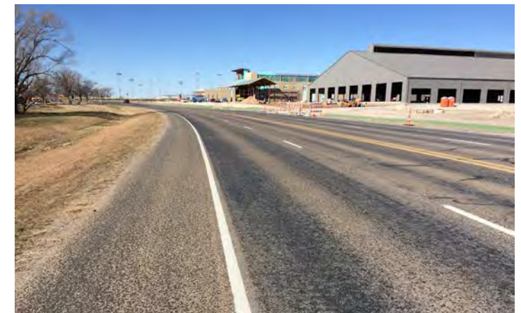
Existing Russell Long Boulevard facing northwest near Ag Sciences Complex
