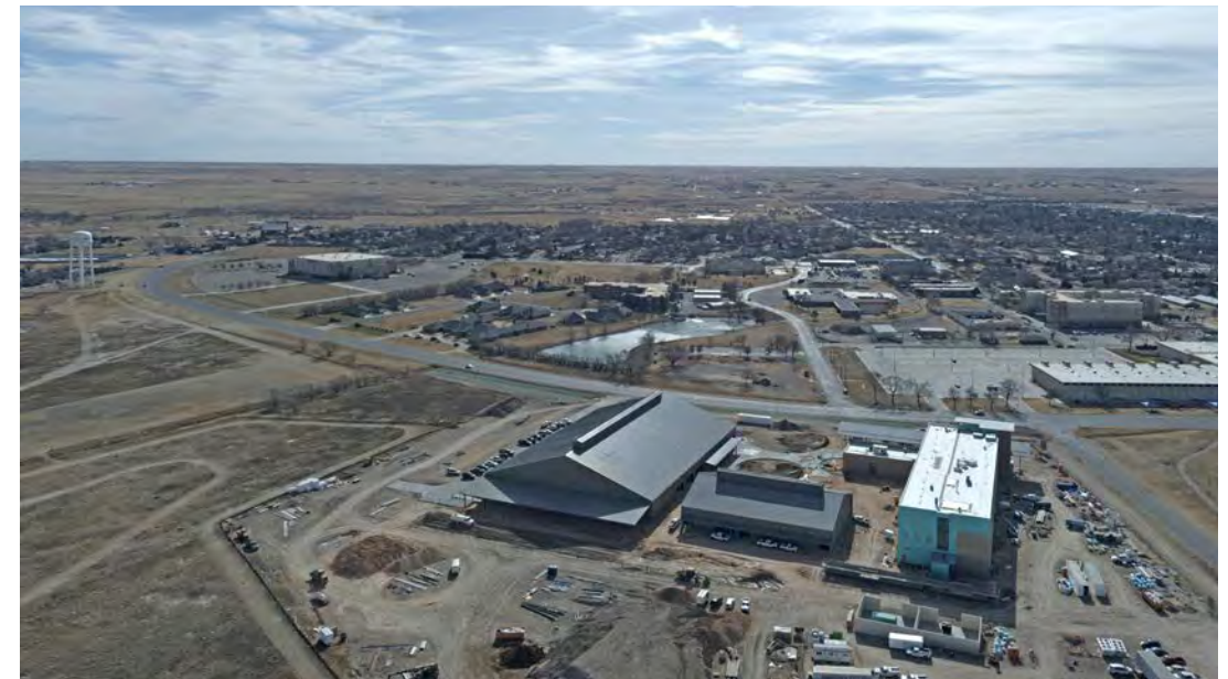
WTAMU Agricultural Sciences Complex under construction on Russell Long Boulevard.
