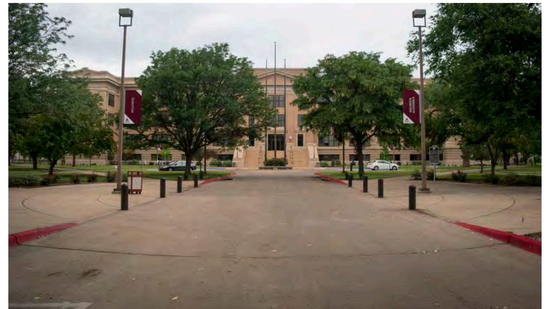
Existing entry drive to Old Main.
