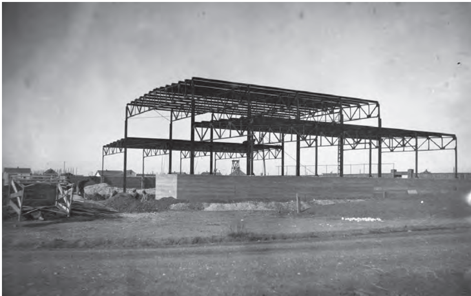
The Box under construction
