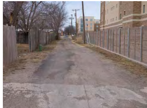
Existing alleyway looking west near 28th
