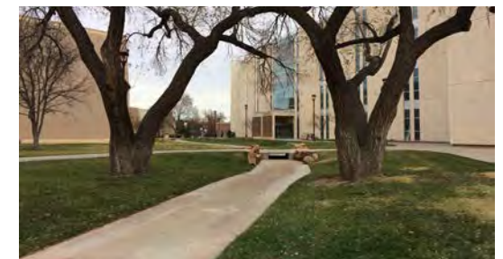
Drainage area between Classroom Center and Sybil B. Harrington. Limited topography in parts of campus have required drainage solutions to alleviate localized ponding.
